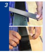
Once the wax has cooled, remove excess FX-Strip material using the CrossFile...
